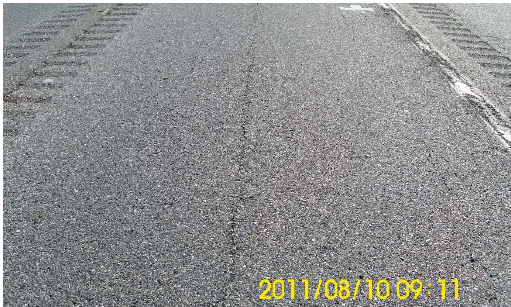
Figure 17. NWP longitudinal cracking on the pavement section in 2011.
