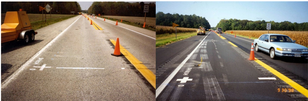
Figure 21. Rumble strips prior to (left) and following (right) the 1998 overlay.
