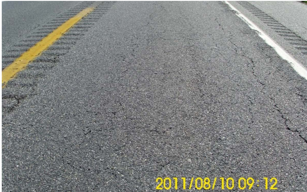
Figure 15. Fatigue cracking on the section in 2011.
